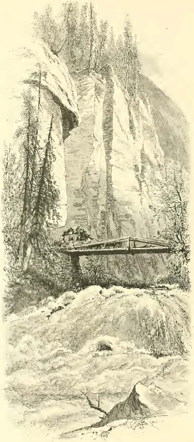
Bridge in Catskill Clove.
